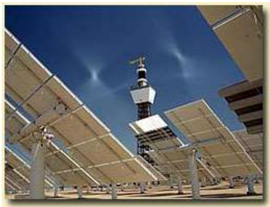
Power tower system
