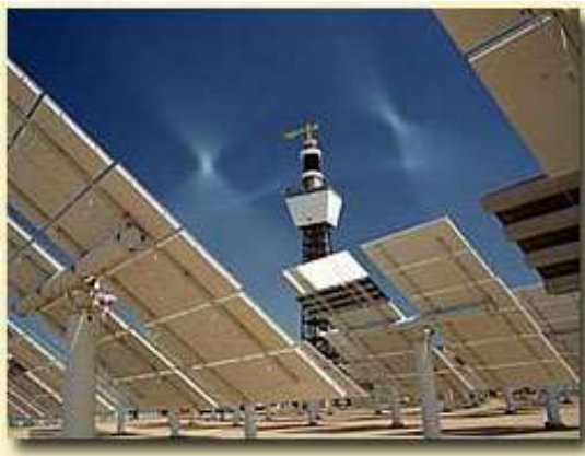
Power tower system
