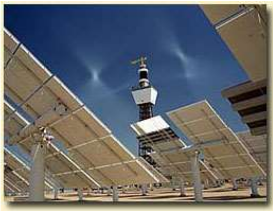
Power tower system
